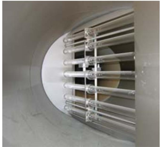
Ultra Violet (UV) lamp bulbs are used for final disinfection in addition to chloramines.
